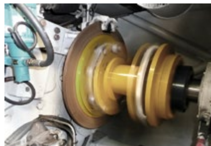
Torque monitoring on wind turbines.
